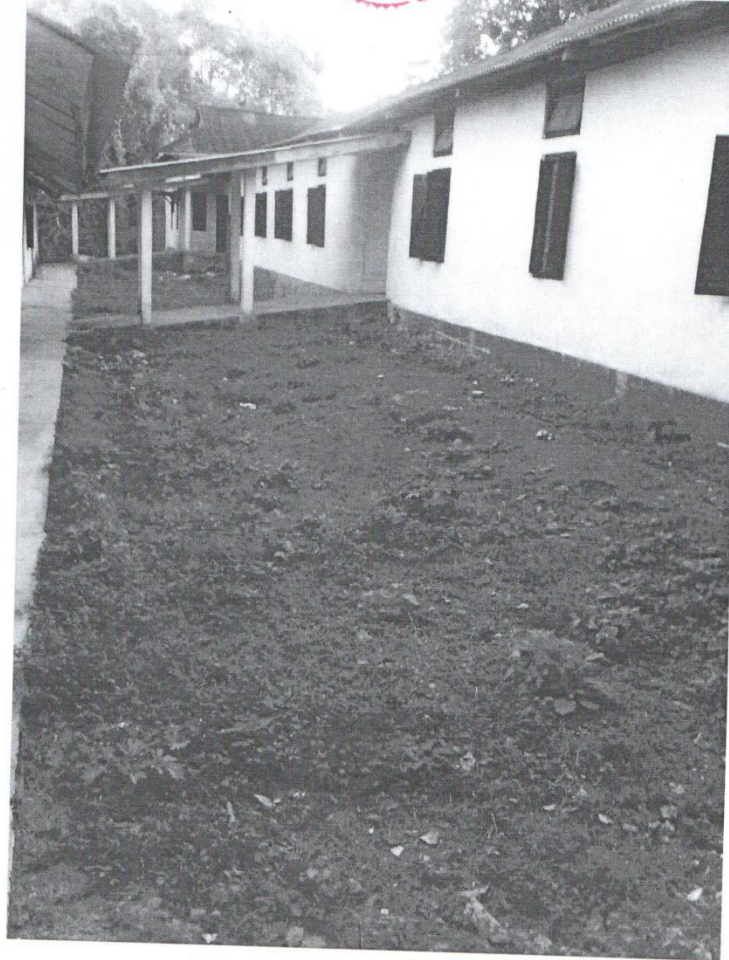
Rear view of the building
